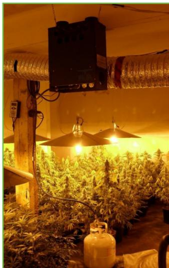
Carbon dioxide burner and propane tanks
